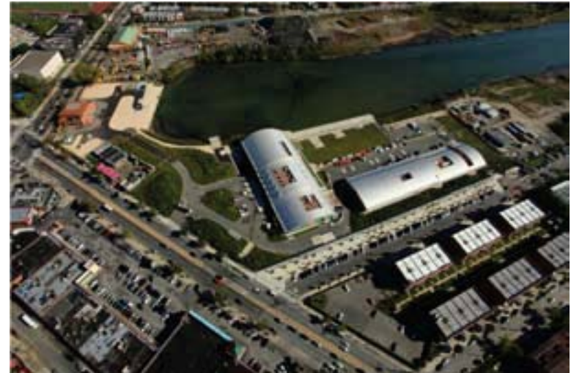
Paerdegat Basin CSO Retention Facility
