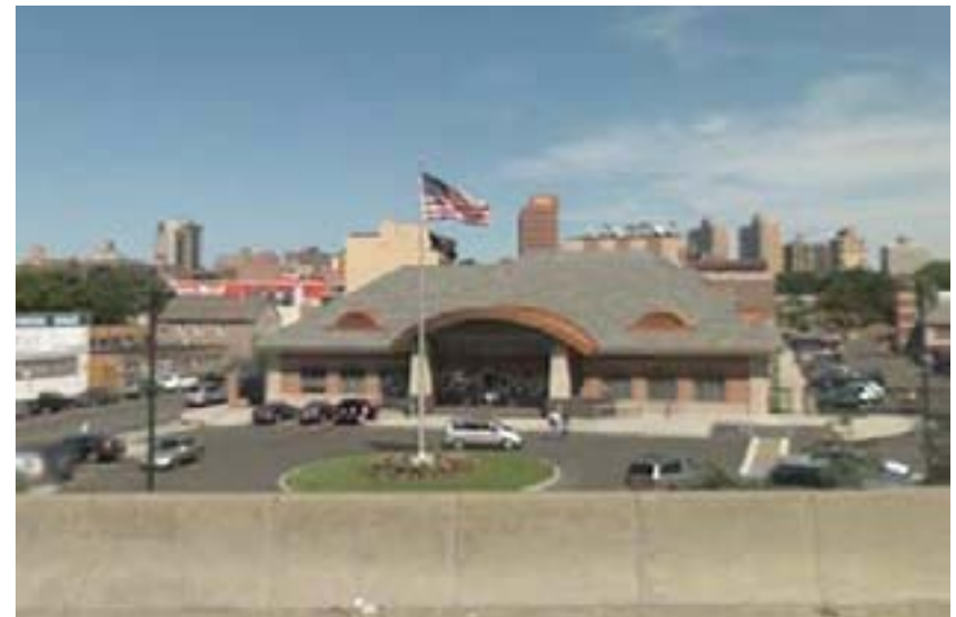
Flushing Bay CSO Retention Facility
